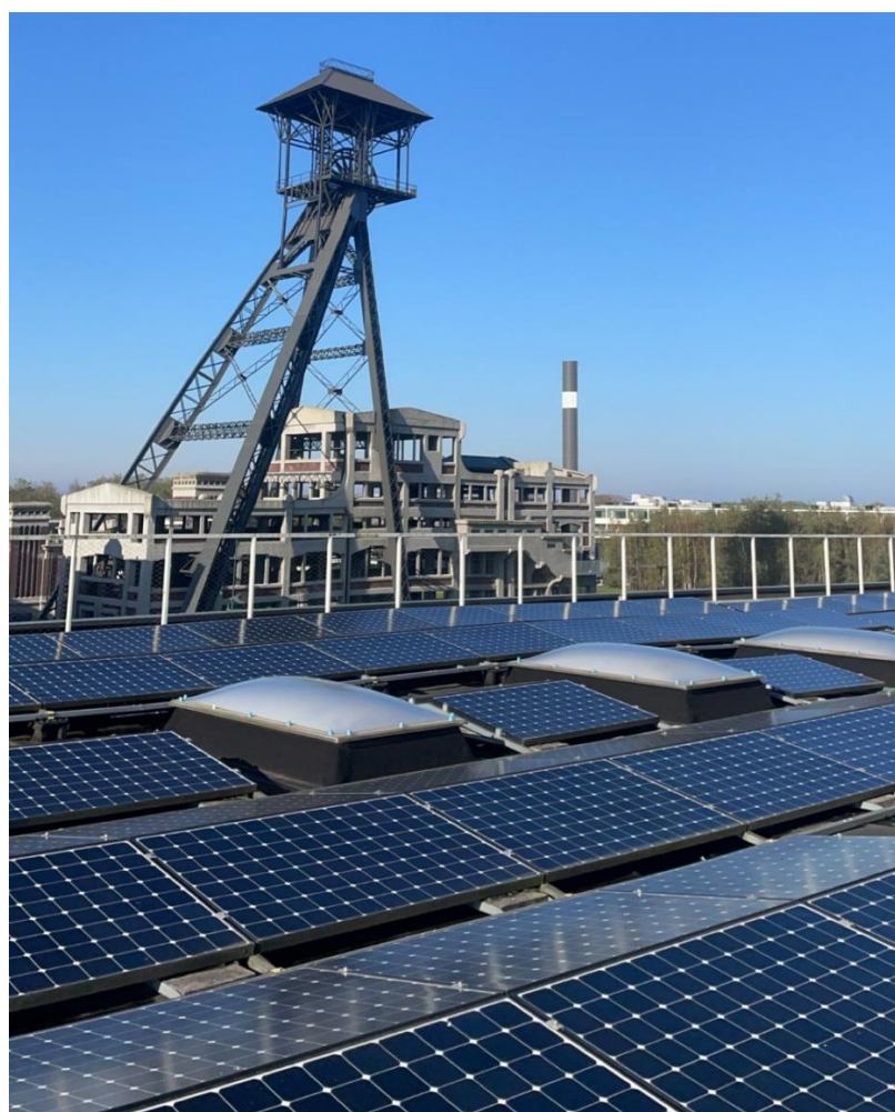
Photo Luca G. (Link) – offers a view from the rooftop next to the solar panels.
